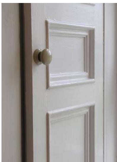
**Right:** At the top of the stairs there is a modification of the opening leading through to the main house . Note the rounded moulding, a decorative detail leading to the upper hall, to the main stair of the farmhouse. This was closed to create a small second bedroom with a door leading through, which is closed off but retained in place.
