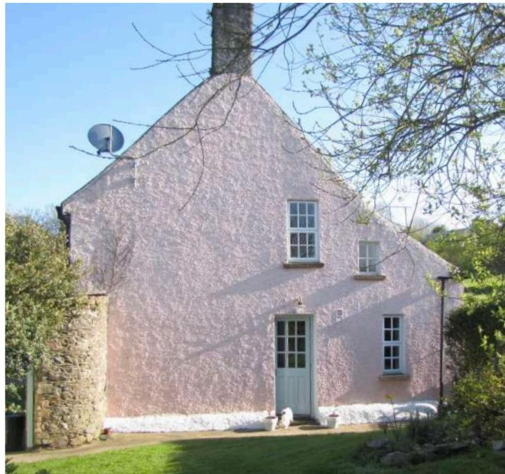
The gable, **left**, has a random pattern of windows. Where the pitch of the roof is less steep, on the right, an extension of the building was added to provide a bathroom. It is also known that The entrance door is recent. Prior to that the only access was through the main farmhouse. It appears that there was previously a window in this location, and that the opening was lowered to give the house an independent access.
