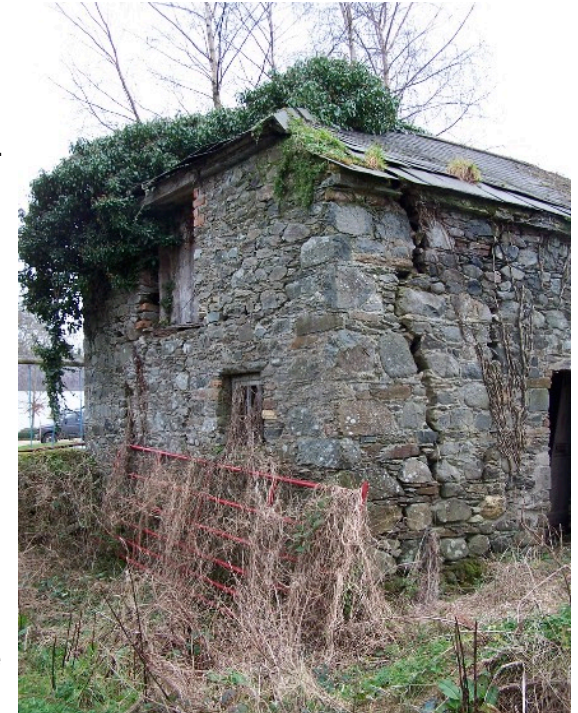
Above: Gable with loft opening above. The major structural crack and the unstable wall beside the loft opening meant that replacement of the roof could be achieved only after the stonework was stabilised.
