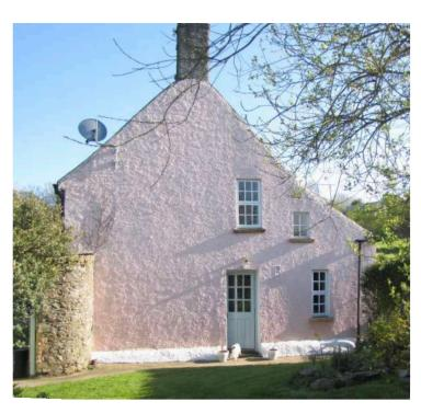
The gable, **left**, has a random pattern of windows. Where the pitch of the roof is less steep, on the right, an extension of the building was added to provide a bathroom. It is also known that The entrance door is recent. Prior to that the only access was through the main farmhouse. It appears that there was previously a window in this location, and that the opening was lowered to give the house an independent access.
